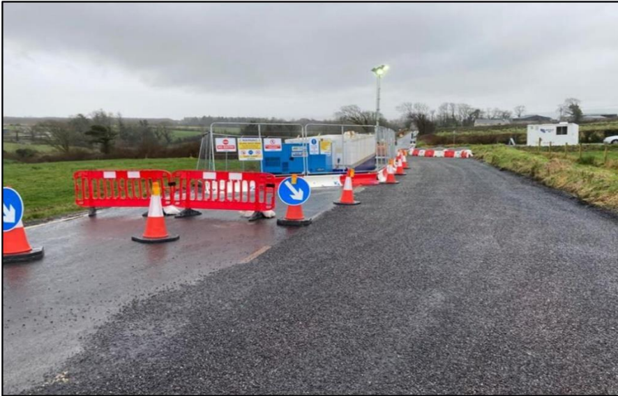
Figure 3-3: Typical Temporary Passing Bay
