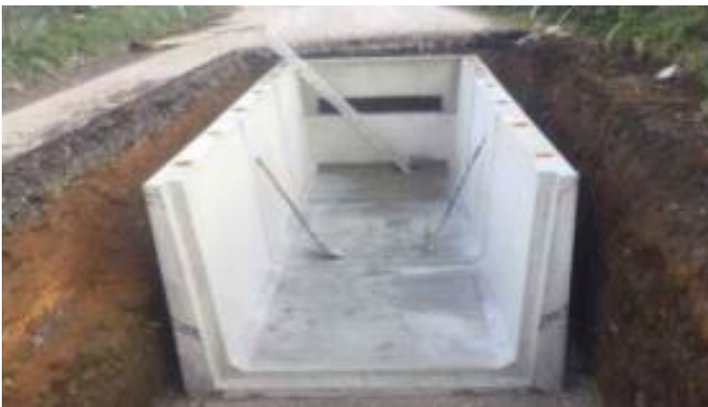
Figure 3-2: Typical joint bay
